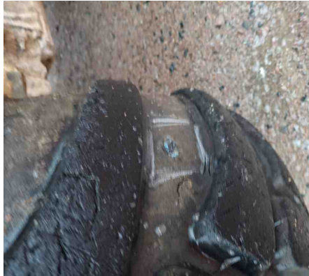
Wheel Position: B1 - Completed Repair
