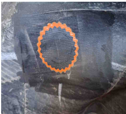
Wheel Position: B3 - Completed Repair
