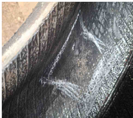
Wheel Position: B4 - Repair Reason
