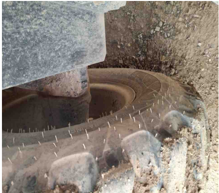
Wheel Position: B2 - Completed Repair
